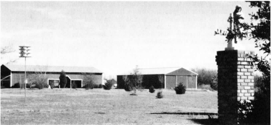
A view of the new but unfinished Carpenter Shop – next to the barn.
