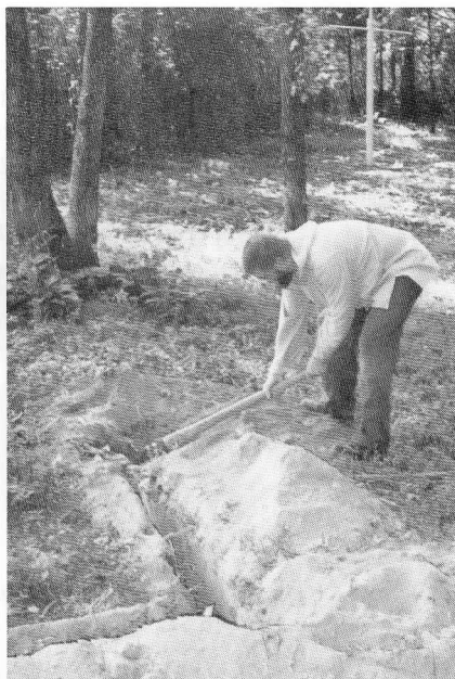
Father Michael, O.S.B. digging a ditch for a new water line..
