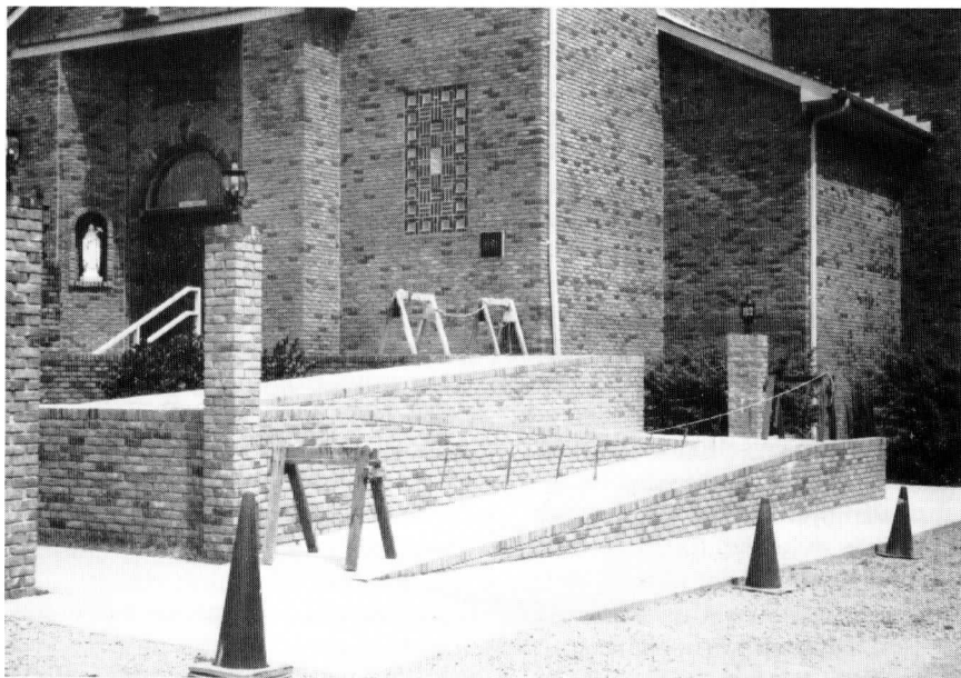
The new (but unfinished) Abbey Church wheelchair ramp.
