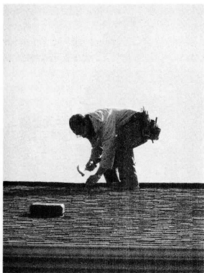
Father Francis repairing the Monastery roof
