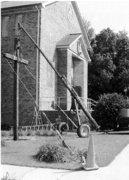
The Cross is set in its place and is made level.
