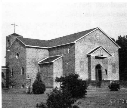
Front view of the Abbey Church looking from the North.
